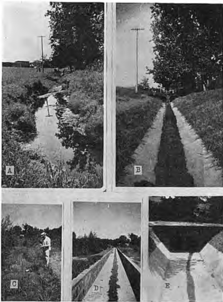
A—Ditch with suitable conditions for mosquito production; B—same ditch as shown in A, but concrete invert has been installed in the bottom, the sides have been sloped and sodded; C—an inspector checking for mosquito breeding in a marshy area; D—same area as shown in C, but after ditch has been constructed and lined with concrete and stone; E—Permanent ditch construction in which small invert for carrying the water during low flow is within the larger concrete ditch.
